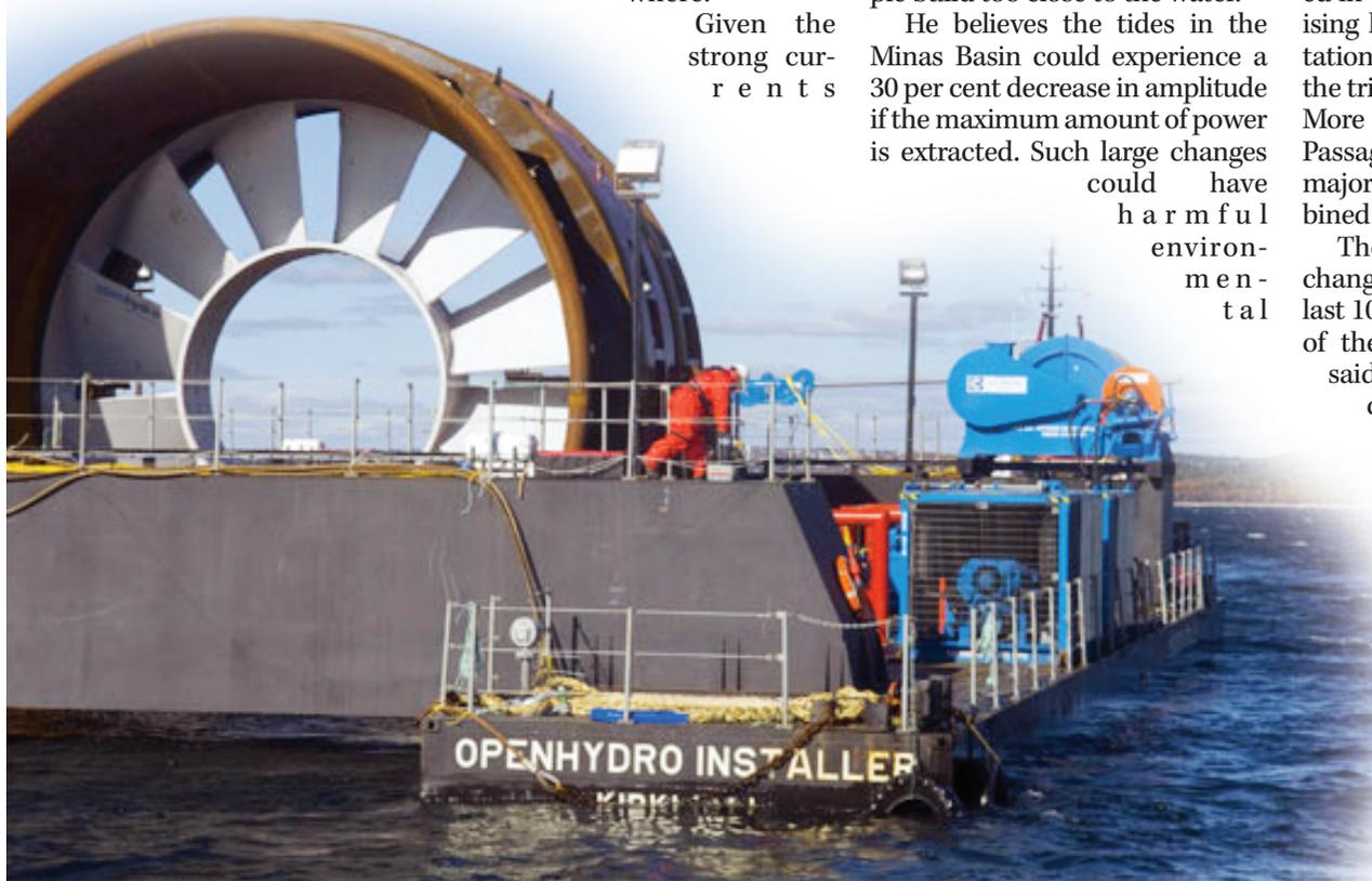
Nova Scotia Power and its tidal technology partner, OpenHydro, successfully deployed the first commercial scale in-stream tidal turbine in the Bay of Fundy in November. The one-megawatt commercial scale turbine reached the Fundy Ocean Research Centre for Energy (FORCE) deployment site in the Minas Passage and is now operational, rotating with the tides, collecting data and producing energy. Submitted
